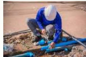
Repaired Pipes ( Environment Friendly)
